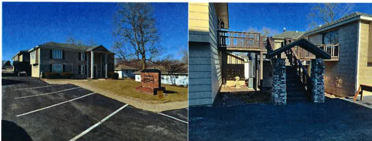
Figure 2 – Site Photos – (L) Front Office Building, (R) Connection Between Front Office Building and Residence/Showroom Building
