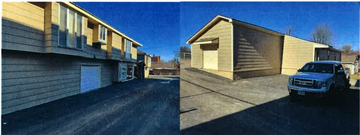
Figure 3 – Site Photos – (L) Central Building with Upstairs Residence and Downstairs Showroom/Workroom, (R) Garage/Storage Building Just Off West End of Central Building
